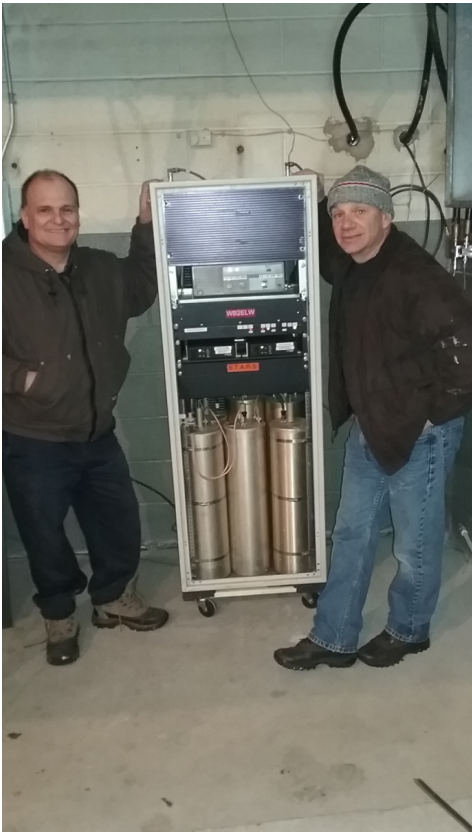
Ken Pokigo, KC2AYK and Mike Fetto, KB2FX after finishing installation
